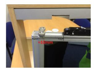
To find the measurement so that you can fit the activator in the top track, measure from the front edge of your door to the front edge of the soft close add on 55mm.
