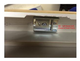
If you measurement from the edge of your door to the start of the soft close was 250mm (Step Two) then the activator should be fitted into the top track 250 + 55mm = 305mm. The activator is fitted from the edge of the activator at 305mm.
